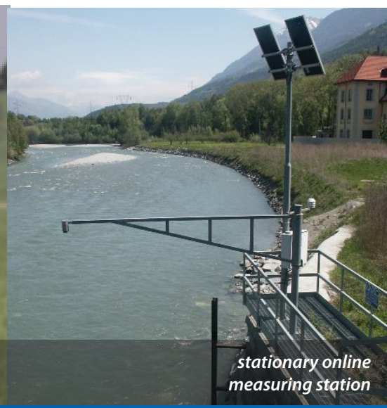
FlashCom/LogCom online-measuring in ground water
